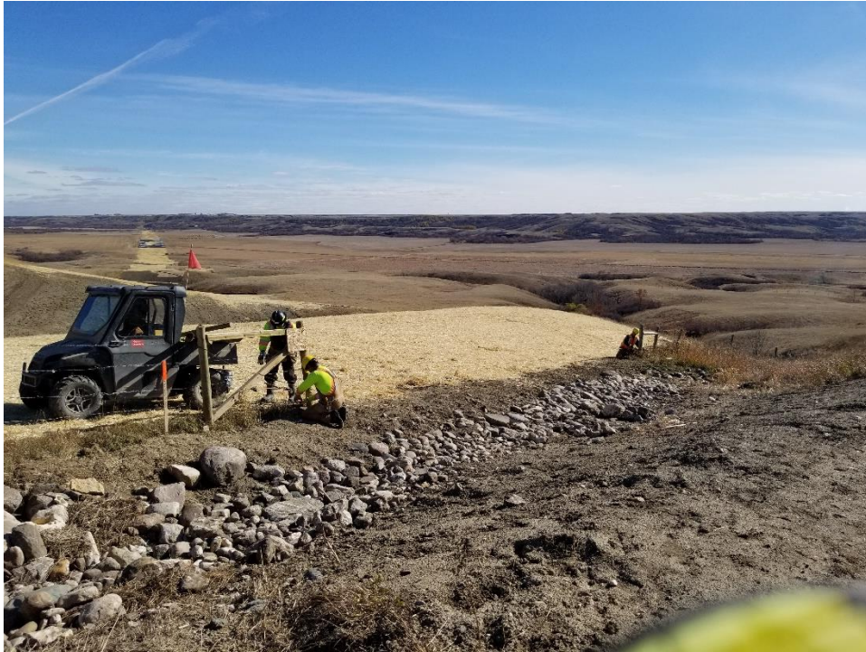
Utility crew installing fence at the Qu'Appelle Valley.
