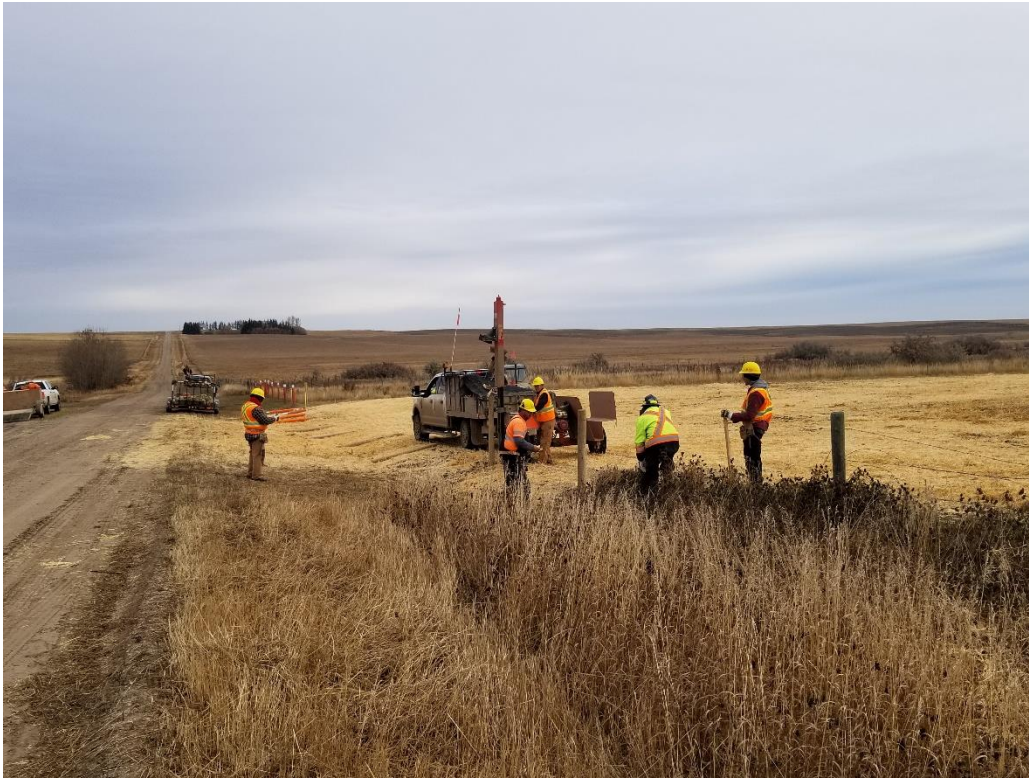
Installing a new fence.
