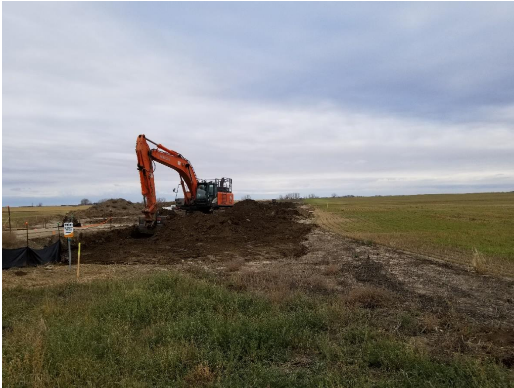
Backfilling a test point.
